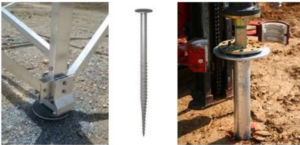
Figure 8: Fondations à visser - Q ENERGY France
