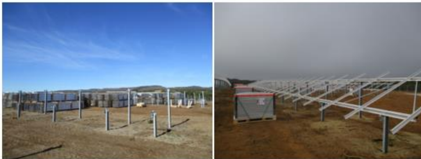
Figure 11: Assemblage des structures - Q ENERGY France
